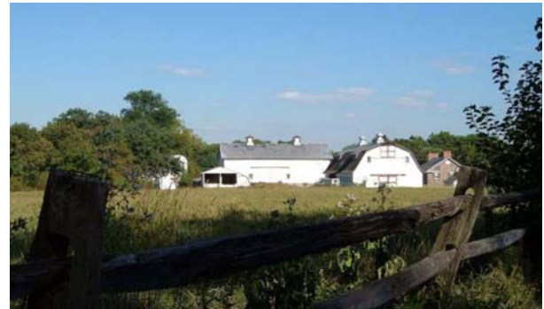
View of Farm Complex from Route 12
